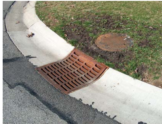
Figure 6. Curb inlet repair site – after.
