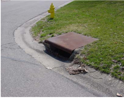
Figure 5. Curb inlet repair site – before.
