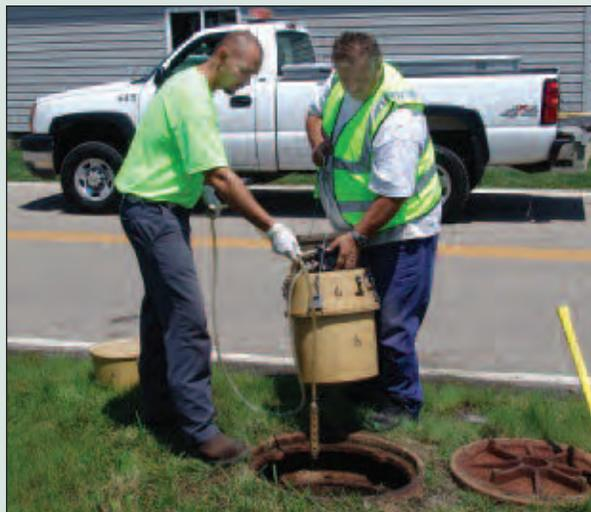
*Wastewater Collection System Crew Members Chris Croucher, left, and Kim Campbell install an industrial waste sampler. The device takes readings every 15 minutes to analyze materials in wastewater flows.*
