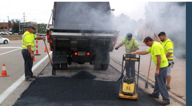
Public Works repairing city road
