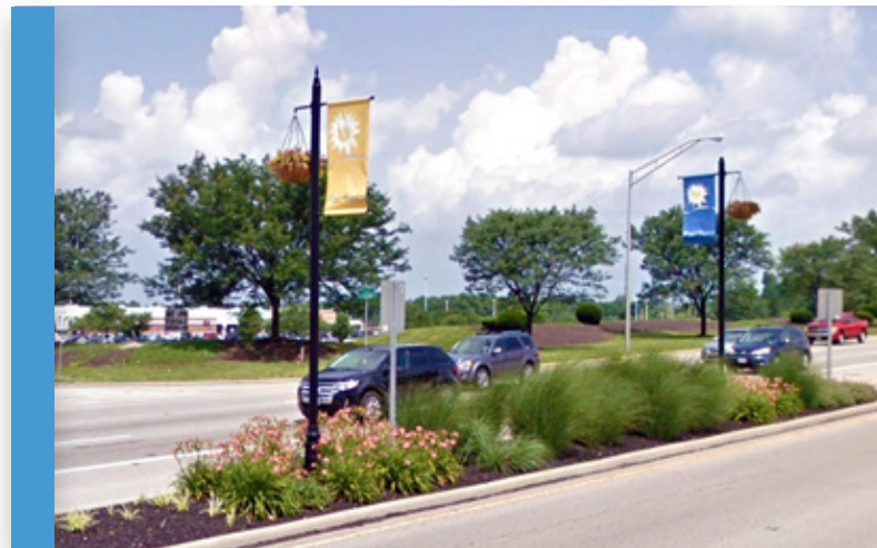
Gateway landscaping and underground utilities on South Gilmore Road
