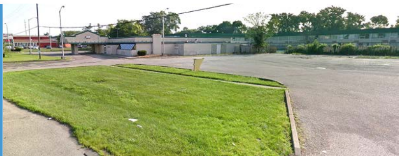
Blighted structure and lot located in the northern section of the Route 4 Corridor
