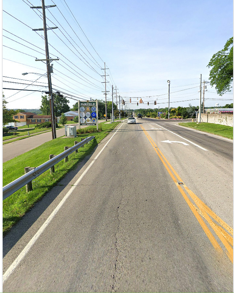
Pleasant Avenue (US 127) north of Hunter Road, looking south
