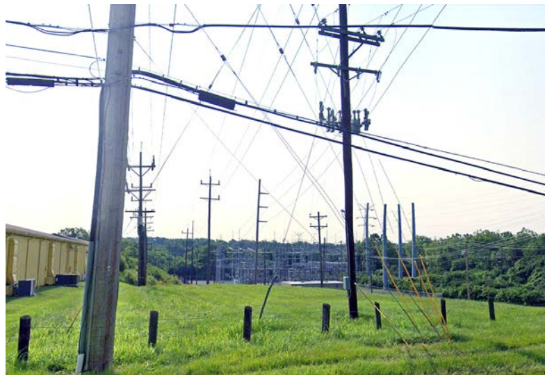
Top: Undeveloped land on the west side of Pleasant Avenue Bottom: Unscreened Duke Energy substation located on Pleasant Avenue
