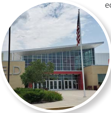
New Fairfield Freshman School constructed in 2018
