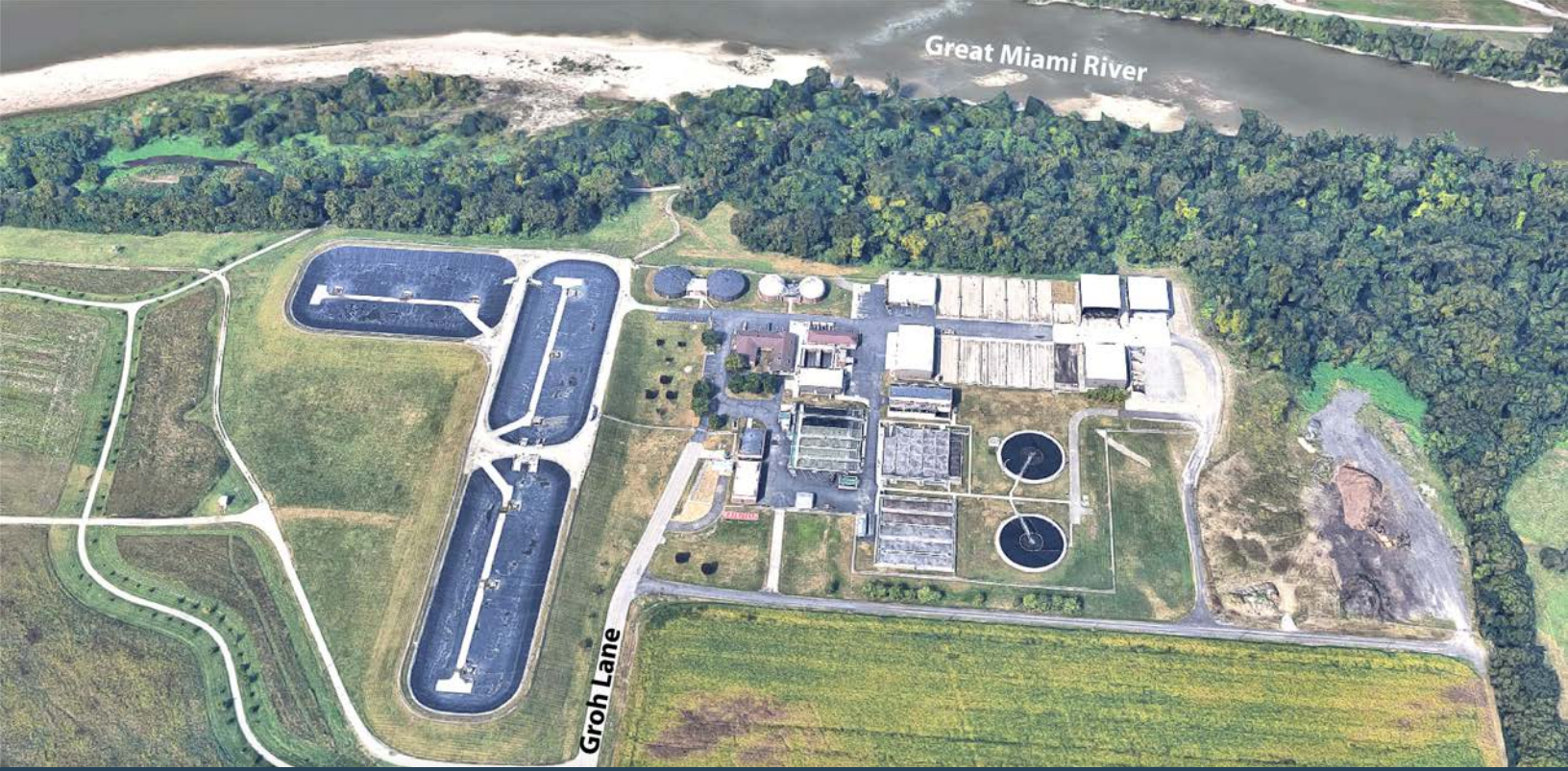
Fairfield Wastewater Treatment Plant on Groh Lane
