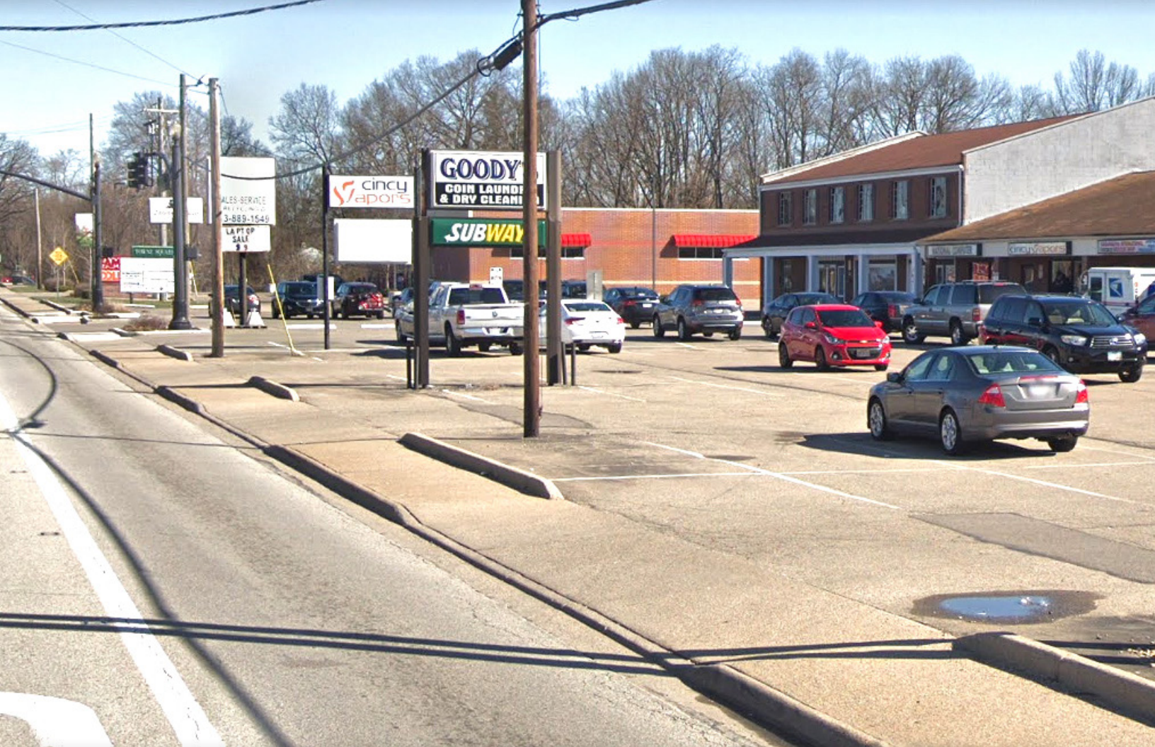
Multiple curb cuts located at an aging commercial strip center on Pleasant Avenue
